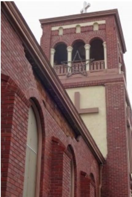
Yeah, that's a whole chunk of facing brick gone. The church is actually not a brick building, it's wood (that's good in earthquake country), with a shell of bricks covering it.
